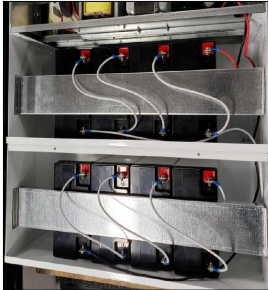
Battery brackets installed on the front
